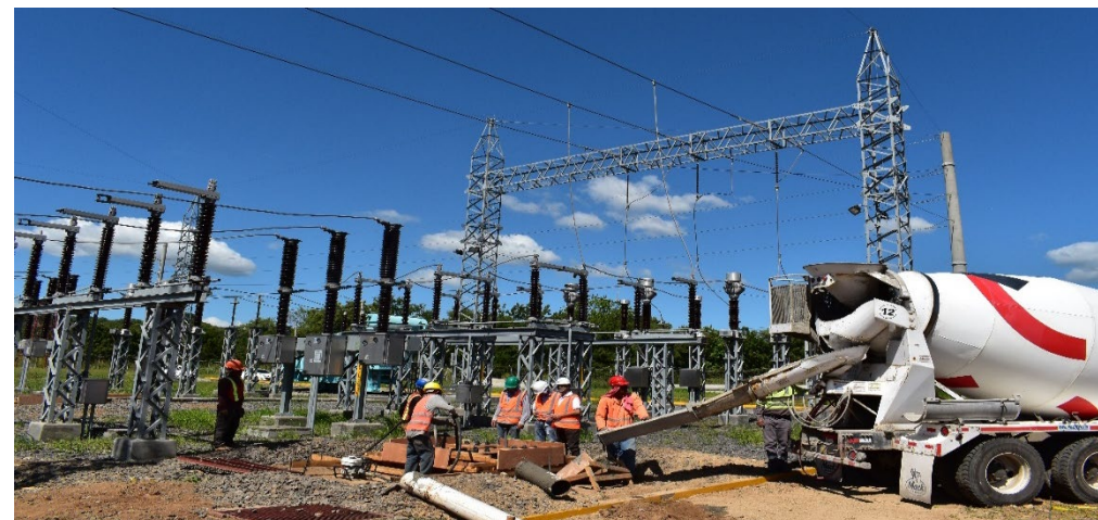
Substation - Gantry Foundation in progress for 138 kV Transmission Line, Nicaragua
