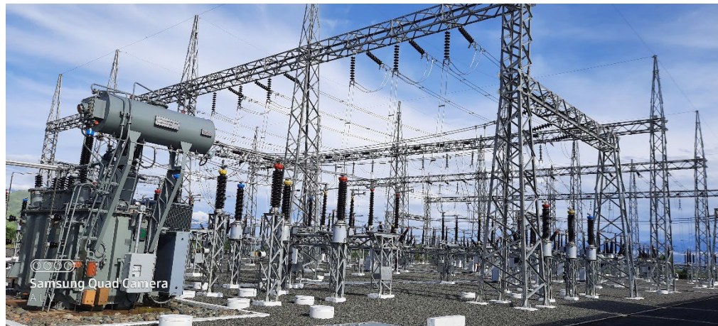
132 kV Air Insulated Substation, Papua New Guinea
