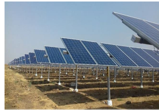
30 MW Tracker Based Installation, Andhra Pradesh
